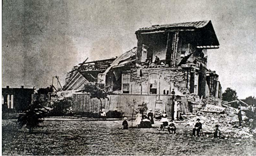
Damage to the Alameda County Courthouse in San Leandro, California, following the 1868 Hayward Earthquake (Source: National Information Service for Earthquake Engineering, EERC, University of California, Berkeley )
