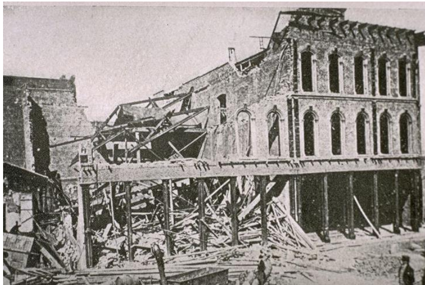
Damage in downtown San Francisco resulting from the 1868 Hayward Earthquake. (Source: National Information Service for Earthquake Engineering, EERC, University of California, Berkeley )
